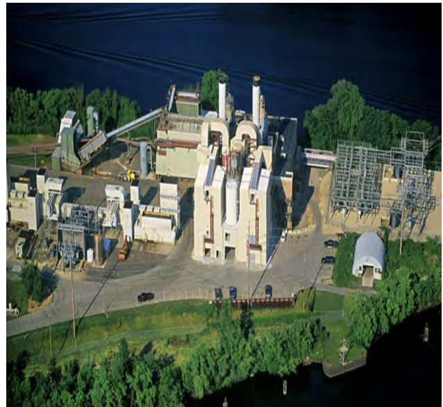
Figure 6-1. Refuse-Derived Fuel Processing Plant
