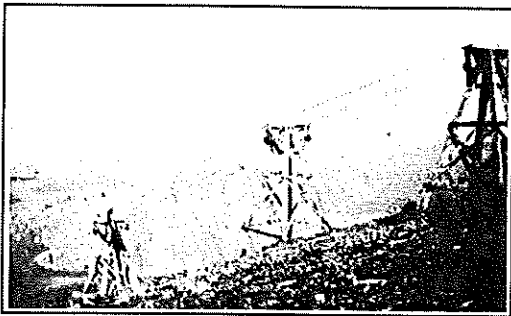
TRAM TOWERS — CABLE TO SEND BUCKETS OF WHEAT DOWN TO STEAMBOATS ON COLUMBIA RIVER AND BACK UP TO BIG BEND PLATEAU WITH LUMBER OR SUPPLIES.
